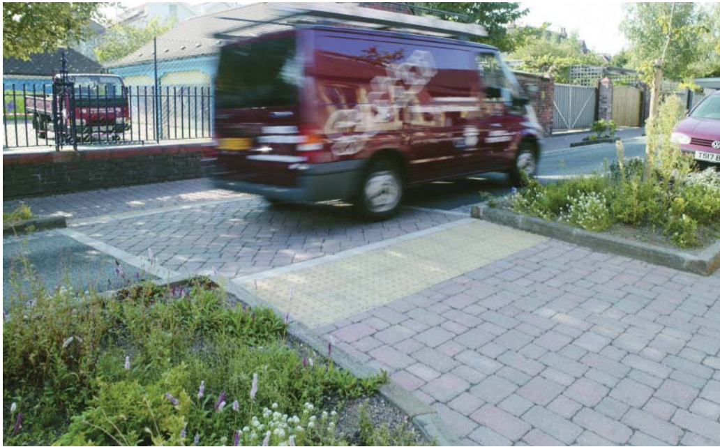
Footpath/carriageway: concrete setts (random course laying pattern, two variations in colour), concrete kerbs and edging
