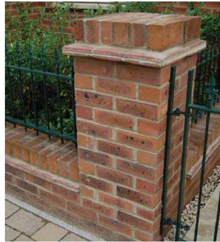
Combined low masonry wall with pillars, railings, coping detail
