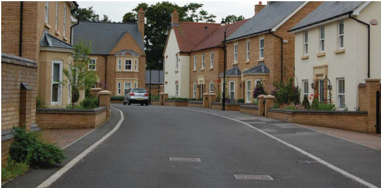
Asphalt road and footpath with contrasting silver grey kerb and edging.
