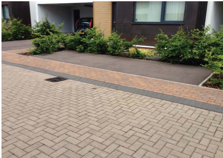
Parking bay: Asphalt; Footpath/carriageway: concrete setts/edging
