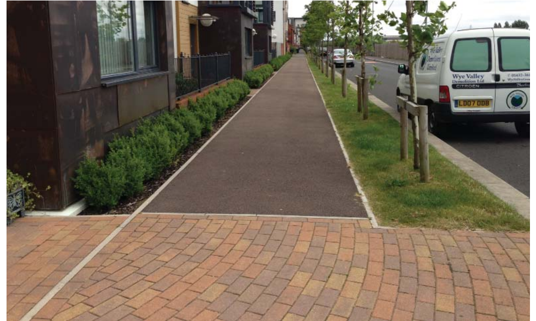
Footpath: Asphalt, concrete setts crossing detail, concrete edging
