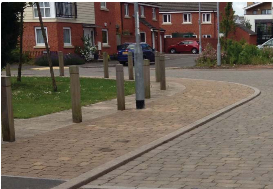
Footpath/carriageway: concrete setts (random course laying pattern, two variations in colour), concrete kerbs and edging
