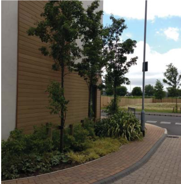
Asphalt road and footpath with contrasting silver grey kerb and edging.
