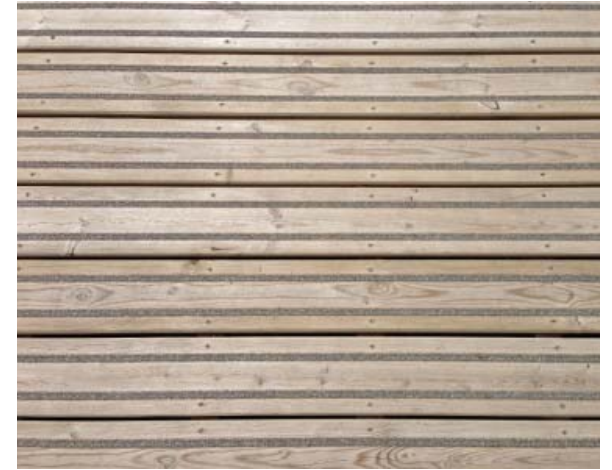
Decking: timber with anti slip feature
