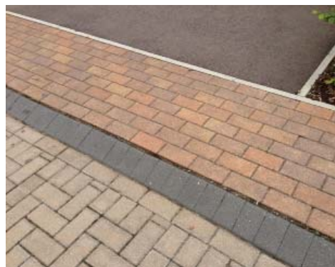
Kerbs/edges: Concrete block kerb half battered
