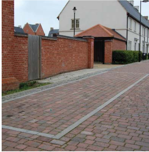
Delineated parking bay: concrete setts
