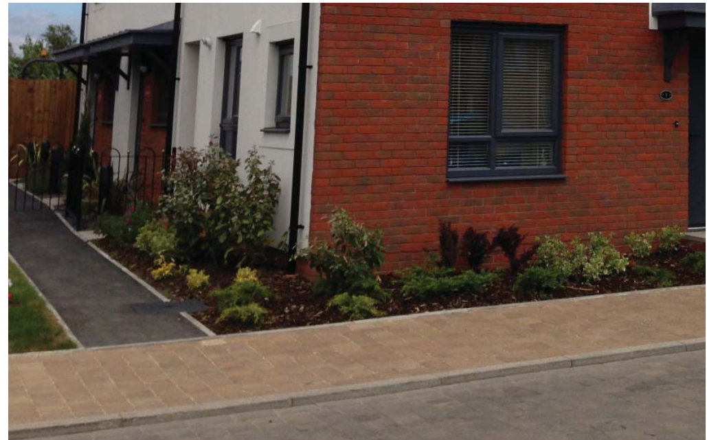
Footpath: Asphalt; concrete setts, concrete edging
