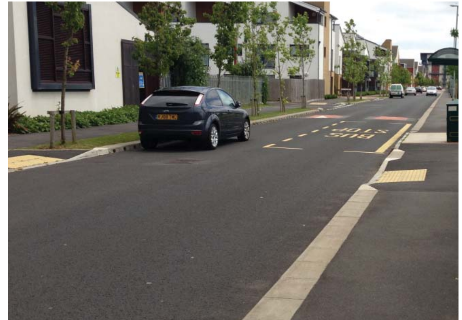
Footpath: Asphalt; concrete setts, concrete edging
